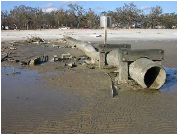
Figure 3. Storm drain for mainland water runoff. This was taken after Hurricane Katrina and depicts shoreline erosion.
