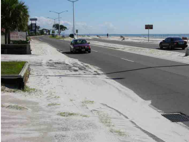
Figure 2. Wind blown beach sand on Highway 90.
