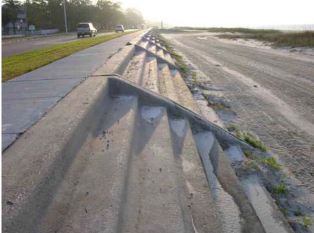
Figure 1. Seawall and the manmade beach
